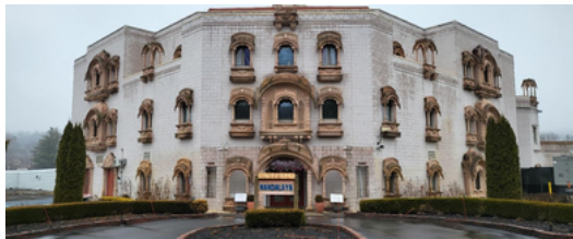
The rear entrance of the Vraj
